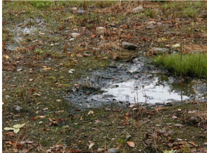
Figure 3: Photos of Failed Septic Systems
