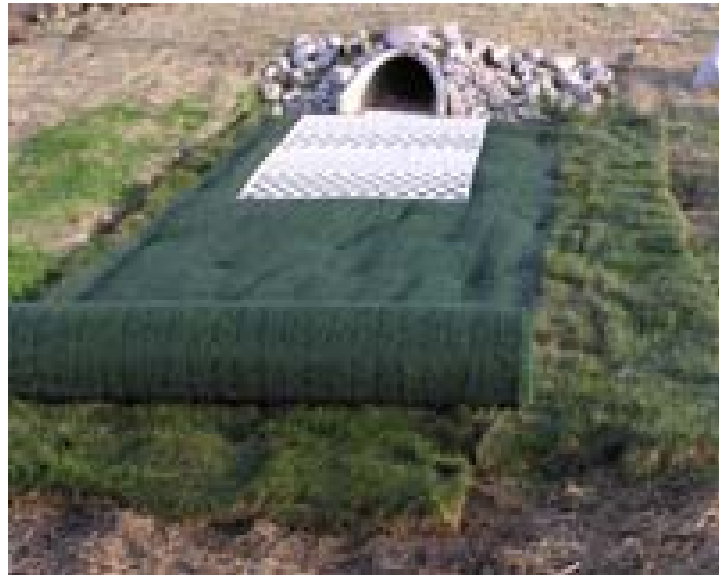
Figure 8: Erosion Control Mat 6
